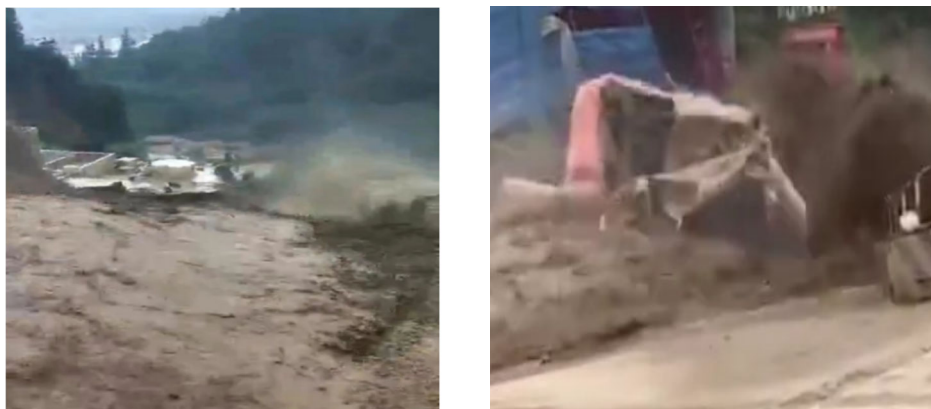
Figure 3. Field pictures of water and mud inrush
