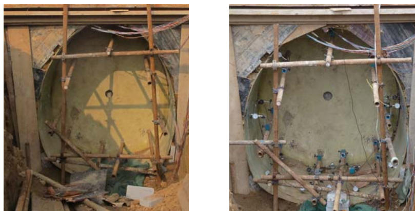
(a) Photo Taken before the Test (b) Photo Taken after the Test
