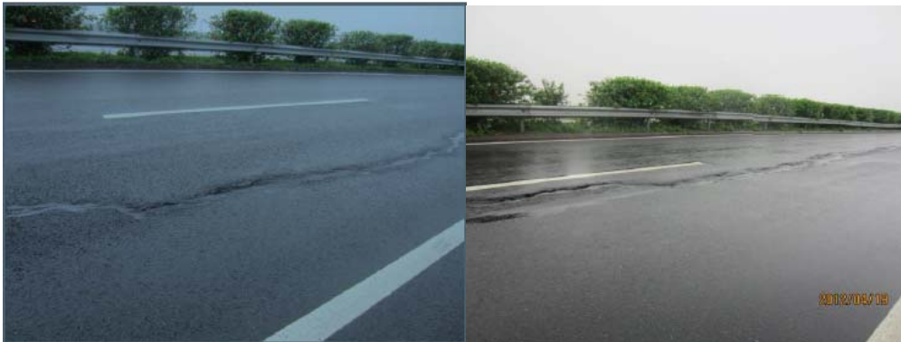
Fig.1 Paving cracking
