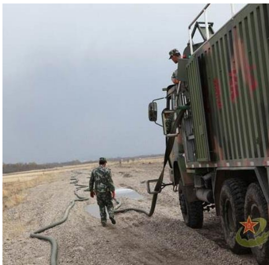
Fig 6. Evacuation and withdrawal of field oil pipeline
