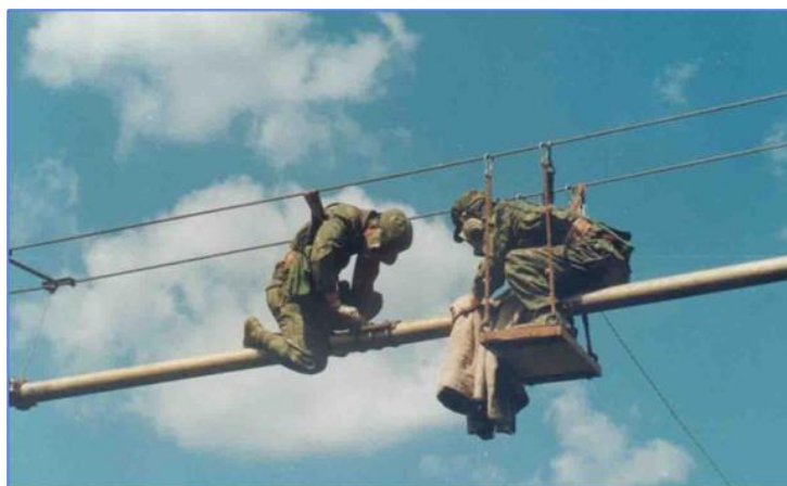
Fig 5. Field oil pipeline inspection and repair
