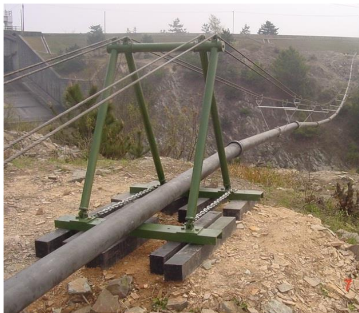
Fig 4. Field pipeline through Canyon
