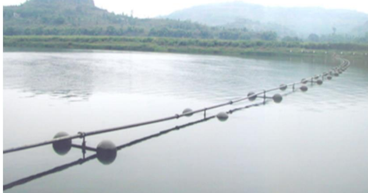
Fig 3. Field pipeline crossing river
