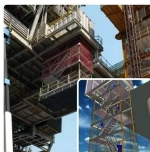
Figure 9. Collapsible remote operating stair system
