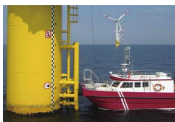
Figure 1. Fixed boarding ladder device
