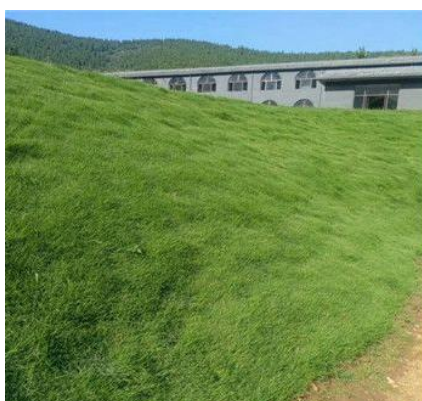
Figure 1. Artificial grass slope protection
