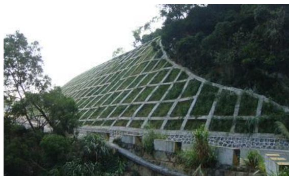
Figure 3. Lattice reinforcement technology
