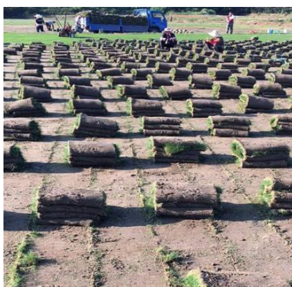
Figure 2. Turf slope protection method
