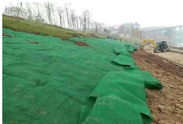
Figure 4. Three-dimensional vegetation net slope protection method
