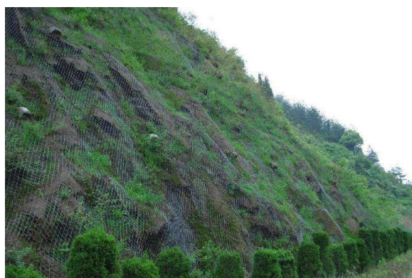
Figure 5. TBS vegetation slope protection technology
