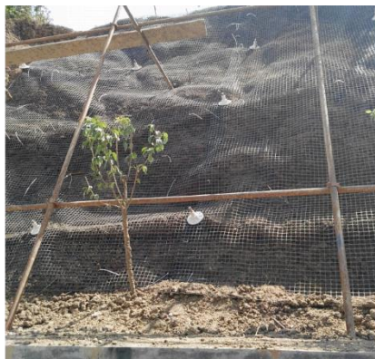
Figure 6. ASE Eco-slope technology
