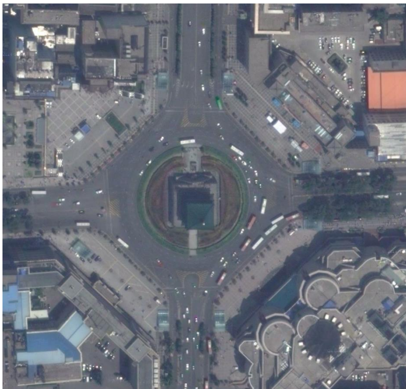
Figure 5. Surrounding environment of xi'an bell tower
