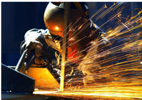
Figure 7. Manual arc welding
