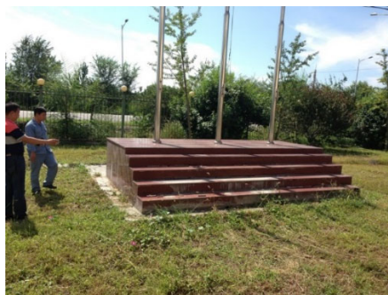
Figure 1. Pipe overlaid flag stand
