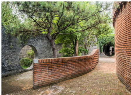
Figure 6. Low wall of small arc bridge
