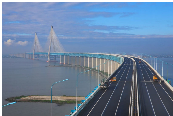
Figure 2. Suzhou-Nantong Yangtze River Highway Bridge
