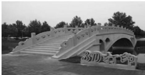
Figure 3. Ma Guowei's team of Hebei University of Technology was built in October 2019 in Tianjin in accordance with the Zhaozhou Bridge 1:2 scaled-down printing
