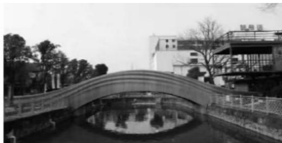
Figure 2. Shanghai Construction Engineering Group completed the 3D printing bridge in Taopu Zhichuang City in 2018
