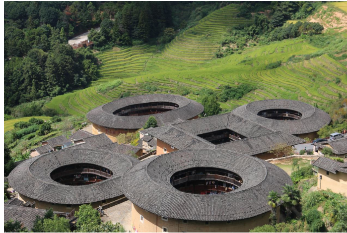
Figure 3. Top view of Tianluokeng Viewing platform
